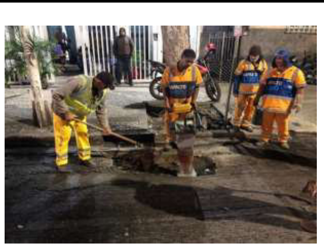
RUA SANTA CLARA REPARO
