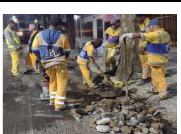
RUA SANTA CLARA REPARO
