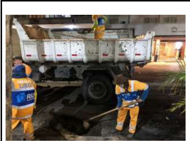
RUA SANTA CLARA REPARO
